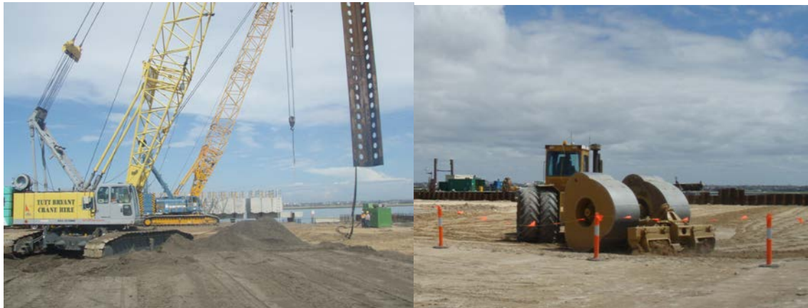
Figure 11: Trial Sheetpile compaction (left) and Dynamic Impact Rolling (right)
