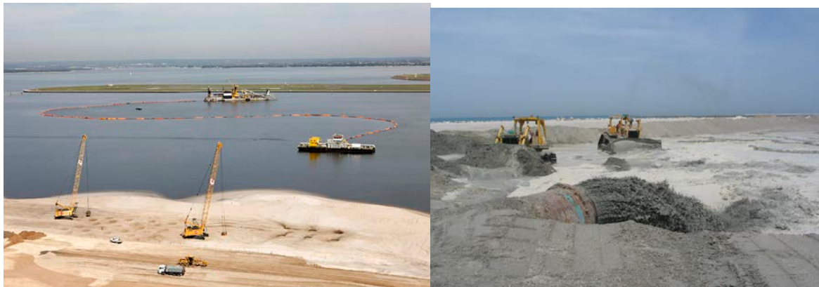
Figure 9: Reclamation activities and discharge lines
