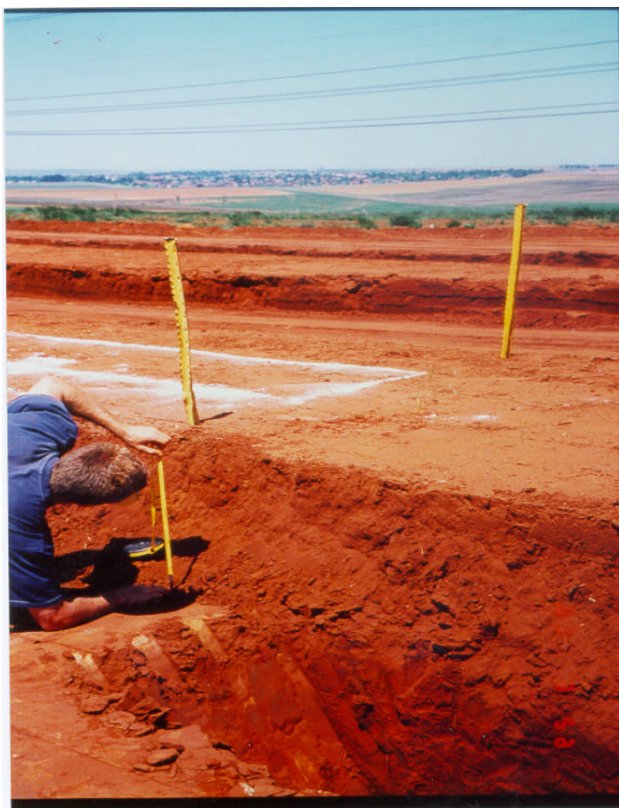
Figure 4: Settlement measurement in 60-pass lane of 25 kJ section
