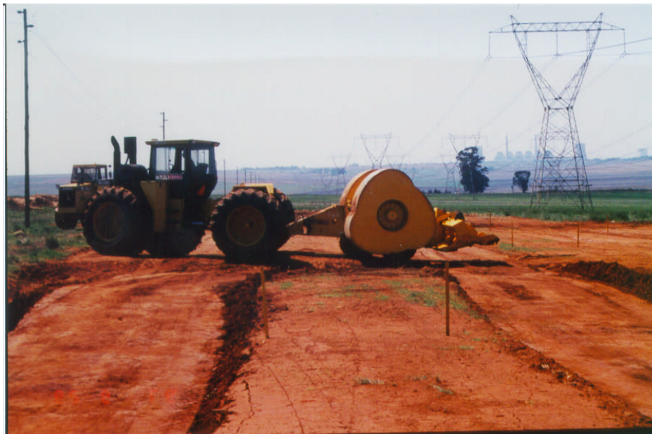
Figure 2: Compaction work in progress with the 3-sided 25 kJ compactor
