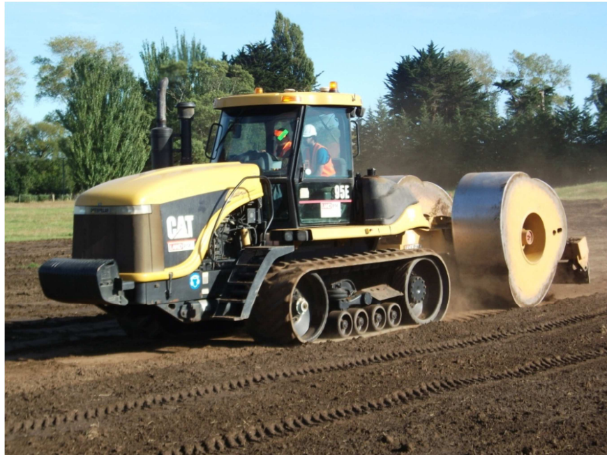
Figure 3 Impact compactor working at the Prestons Subdivision
