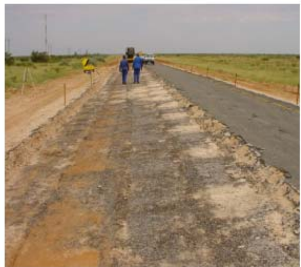
Figure 7. Trial section during the first 5 passes and after 30 passes.
