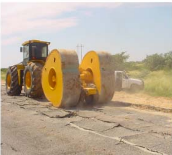
Figure 7. Trial section during the first 5 passes and after 30 passes.
