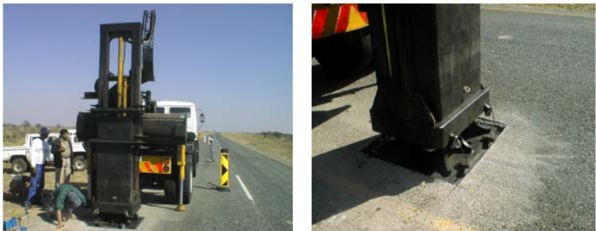
Figure 6. Landpac mini dynamic compactor on the Jwaneng – Sekoma site.
